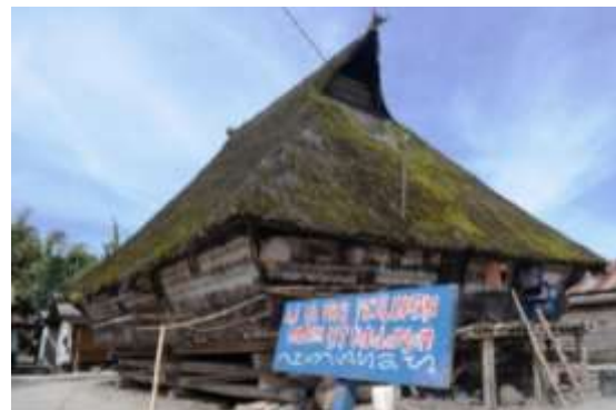
Figure 4. One of the 100-year-old Karo Traditional Houses in Dokan Village
