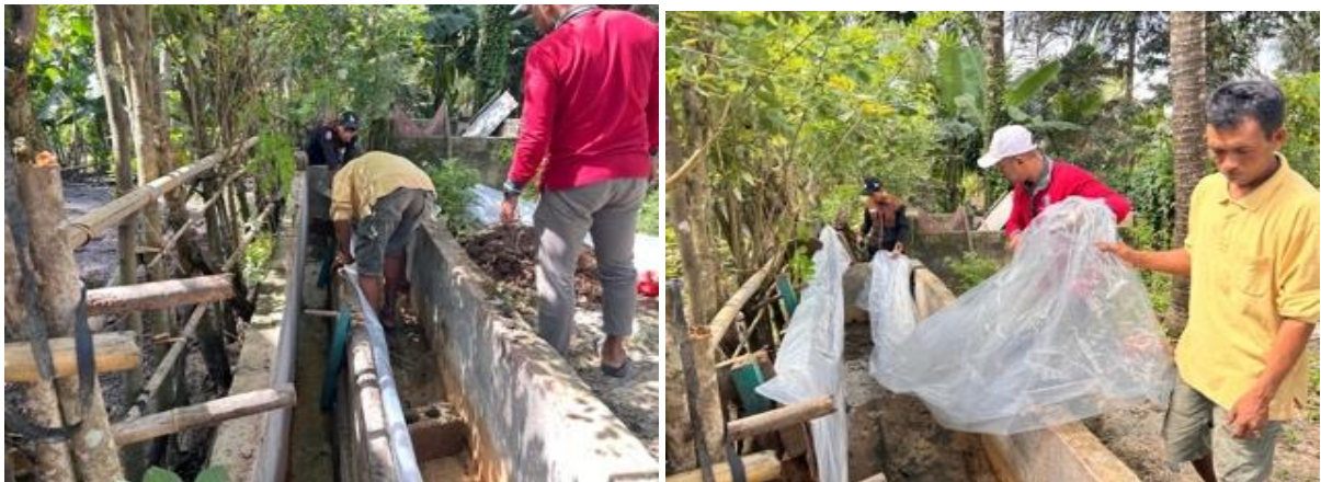
Figure 3. Digester Installation
