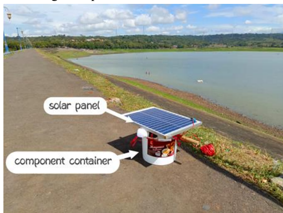
Figure 4. Condition of finished solar panels
