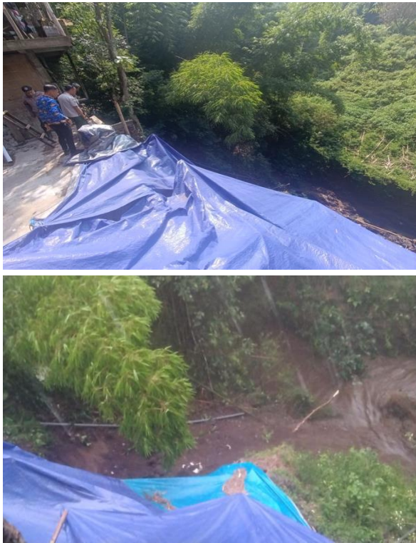
Figure 4. Tarpaulin sheets provided by BPBD are used to prevent soil erosion caused by rainfall (source: personal documentation)
